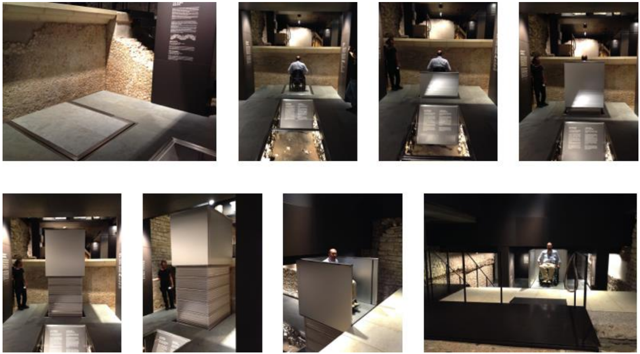
Figure 4. The internal platform lift
